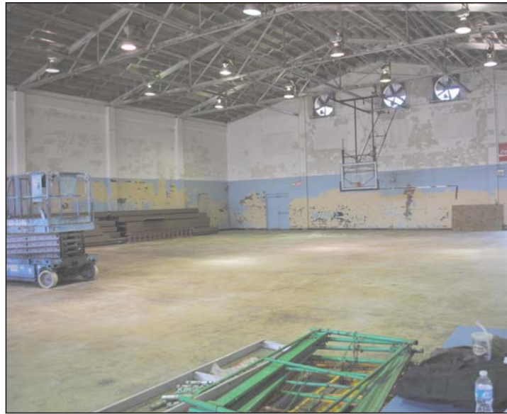
The Gym at The Dream Center, a work in progress
